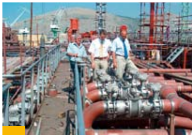
Inspection of prefabricated products after installation
